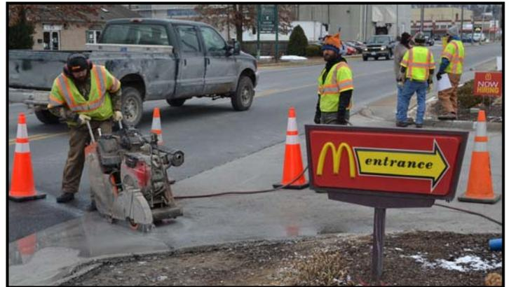
The system our employees installed is not a typical drop inlet that channels stormwater to the river. It's an environmentally friendly technique that collects the stormwater and sends it underground where it will help replenish the water table. A similar method was used at Generations Park and at a problem area on East College Street. The new system will back up during a major thunderstorm, but most rains will readily disappear underground.
